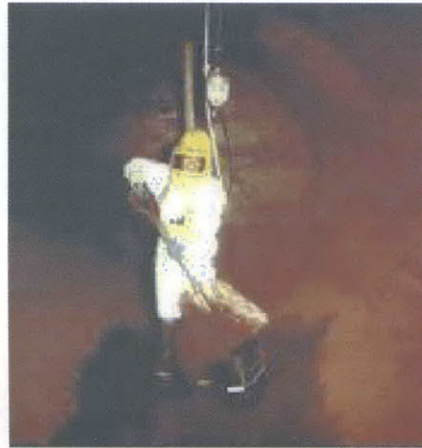
Rehabilitation of a corroded fuel tank
