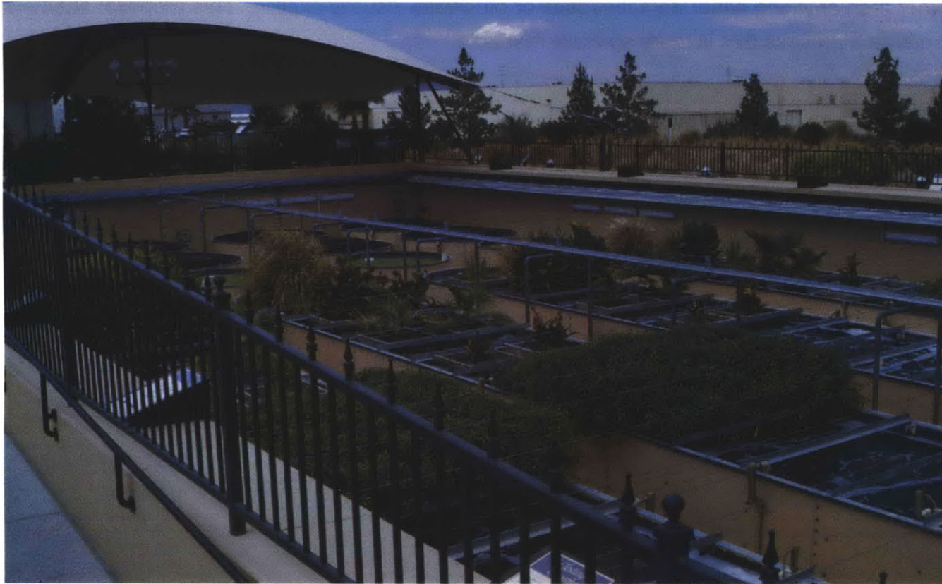
Living Machine Wastewater Treatment Plant, Arizona.
