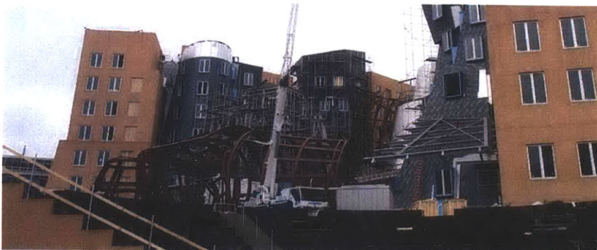
Figure 2.22 MIT Stata Center under construction, Frank Gehry
