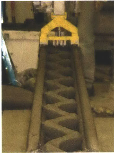
Figure 2.17 (Above) Contour Crafting, automating construction of whole structures and structural elements by Behrokh Khoshnevis USC ( http://www.contourcrafting.org ). Detail of wall structure created with Contour Crafting. Detail of Contour Crafting nozzle in action
