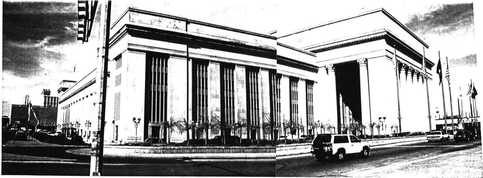
Figure 2.13 View of 30th Street Station
