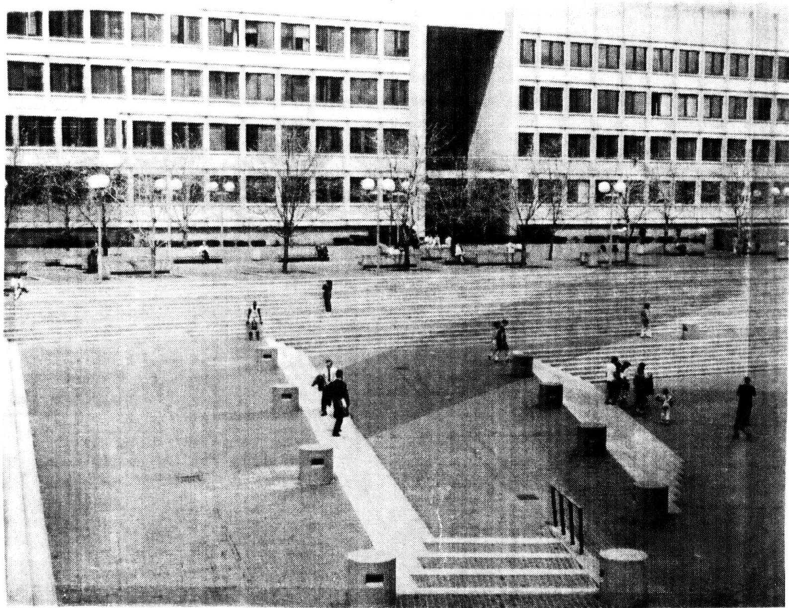
The plaza - in front of the Federal building.
