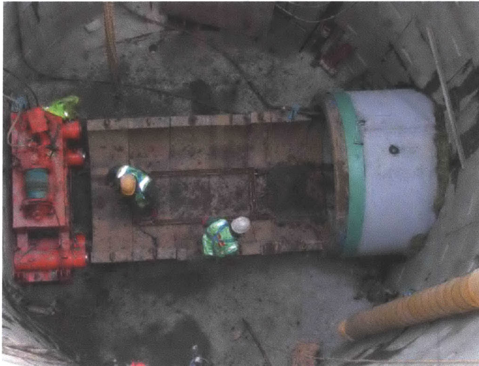
Figure 6-3: Pipe jacking process (Vorster, 2005)
