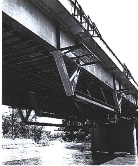
Figure 13: SAVA system installed on the Walnut Creek Bridge [22]
