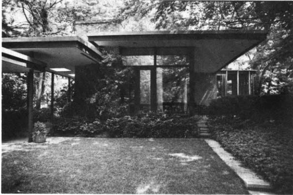
Figure 3.27 (left) Overhangs on this residence are longest on the south and east sides, and are white underneath. (right) Jose Luis Sert's housing for Harvard, showing vertical, manually operated louvers on the western facade.
