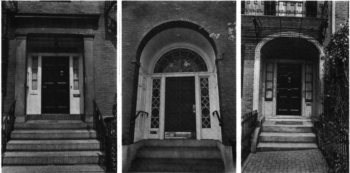
Figure 2.13 The evolution of the transom with side-lights; from rectangular to semicircular to elliptical. (Beacon Hill)
