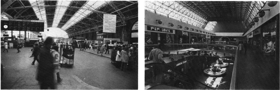
Figure 3.14 London's railway stations and America's shopping malls (Chestnut Hill, Ma., in this photo) exemplify the use of skylighting in public spaces.
