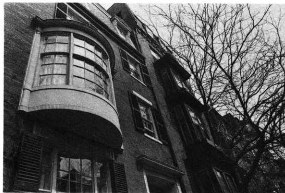
Figure 2.7 (left) These shutters fold back into the reveals of the window. They are also adjustable like venetian blinds. (right) Both types of bays are seen on this facade on Boston's Beacon Hill.
