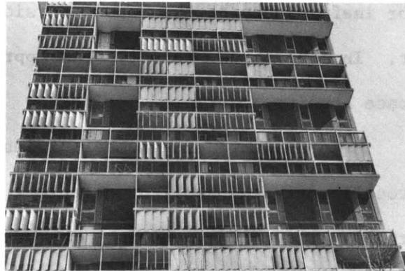
Figure 3.27 (left) Overhangs on this residence are longest on the south and east sides, and are white underneath. (right) Jose Luis Sert's housing for Harvard, showing vertical, manually operated louvers on the western facade.
