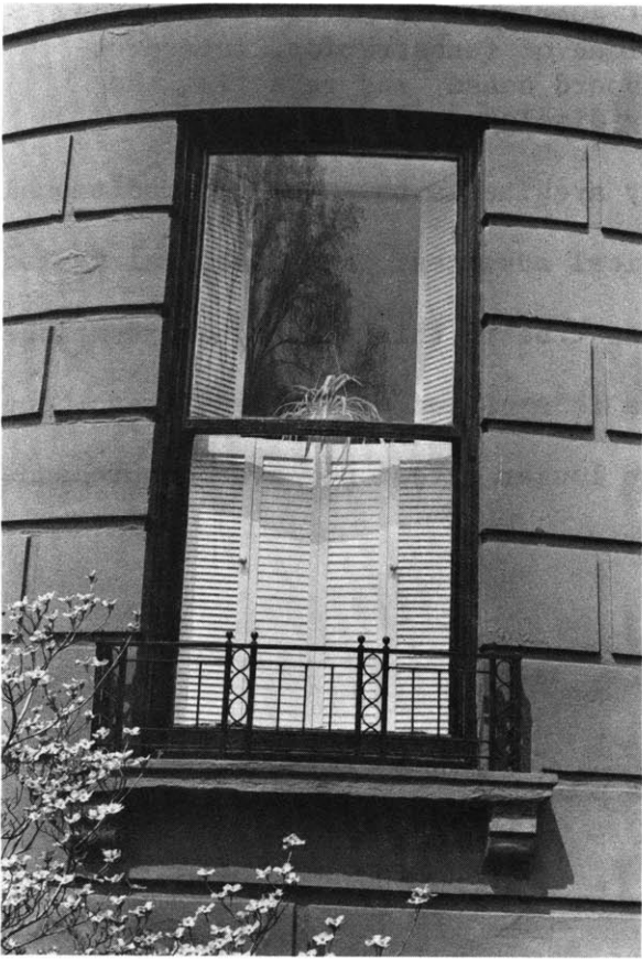
Figure 2.7 (left) These shutters fold back into the reveals of the window. They are also adjustable like venetian blinds. (right) Both types of bays are seen on this facade on Boston's Beacon Hill.
