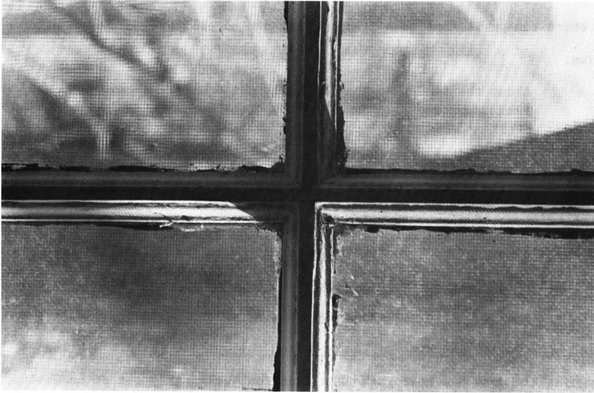
Figure 3.16 "Molded" mullions and muntins also serve to grade the brightness from the window to the wall.
