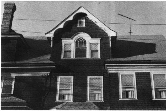
Figure 2.12 (left) A late-19th century Palladian window in Brookline, Massachusetts. Note also the diamond-shaped lights. (right) The windows in Faneuil Hall (1742) take up nearly 50% of the wall area: this is the stairway.
