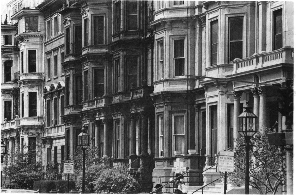
Figure 3.6 Bays on Boston's Commonwealth Avenue.
