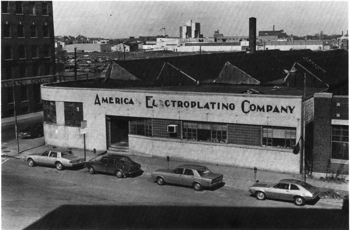
Figure 3.10 Northlights on a Cambridge factory.
