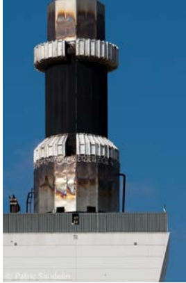
Figure 1.2: Solar Two receiver after the three years of operation (DOE & Sandia, 1998).
