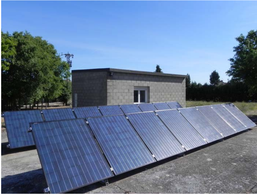
Figure 4.3: Laboratory building and PV/T array.
