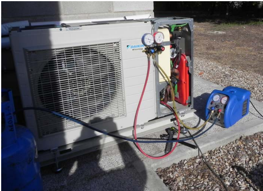
Figure 8.29: Heat pump's refrigerant refill operation.
