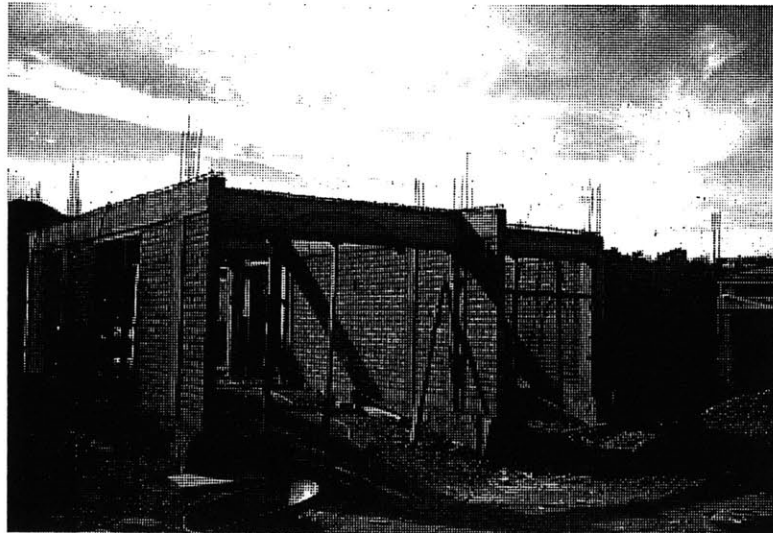
Building under Construction in Mulegé
