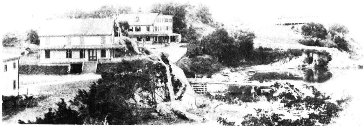
Early view of the site showing the Resort at Chapel Rock Looking west from Rock showing hotel, dance hall and residence
