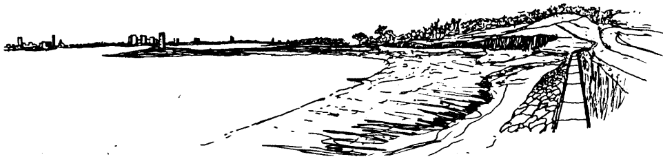
View north towards jetty from approaching road with Boston in the background
