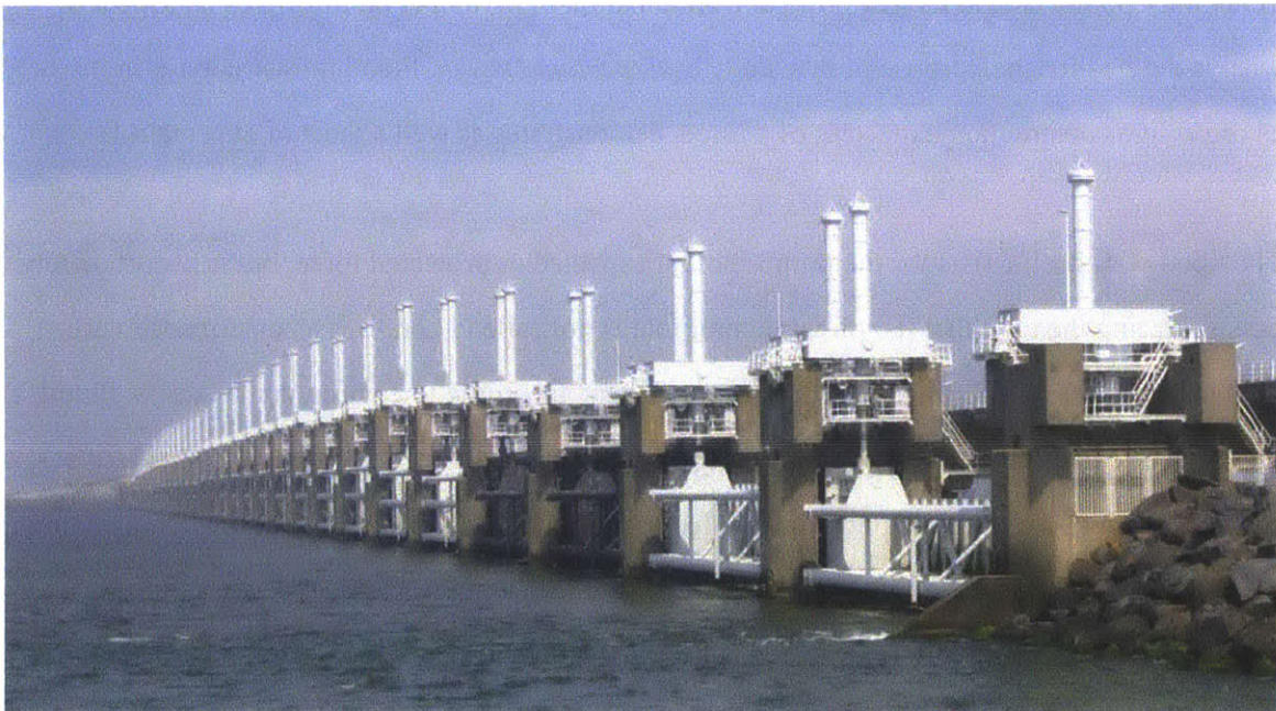
Flood infrastructure as inspiration for Expectant Design. Oosterscheldekering (Eastern Scheldt ) storm surge barrier in the Netherlands. Image: Vladimír Šiman.
