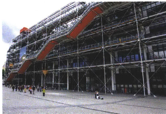
The Pompidou Centre's externalization of systems in an attempt to free up and neutralize the interior, in preparation for multiple uses. Image: Edal Anton Lefrov.
