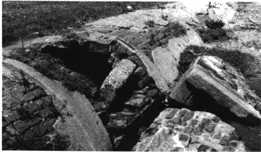
Outfall Pipe near its Discharge Point
