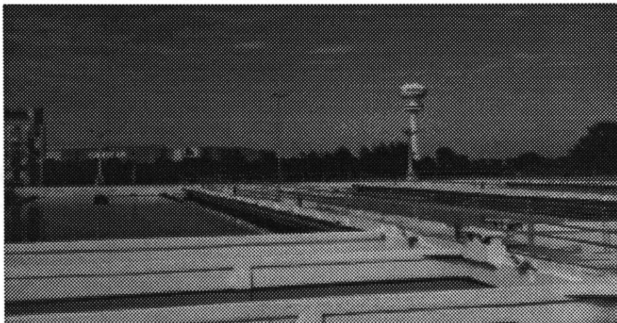
The La Plata System's Water Treatment Plant
