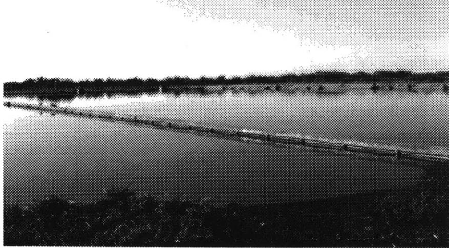
La Plata System Wastewater Treatment Lagoons
