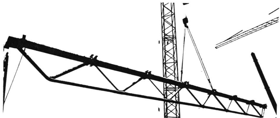
[42] The Centre Pompidou steel lattice girder
