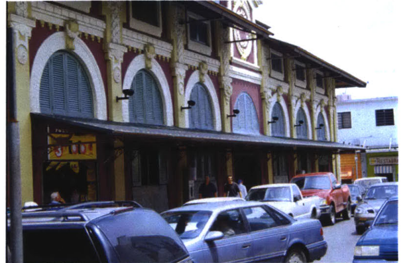
fig. 33 Market, Santurce. Market hall exterior.
