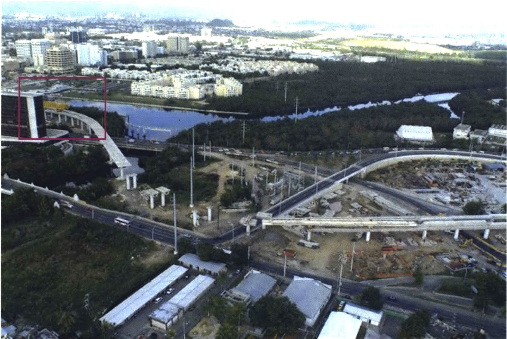
fig. 105 View of site. Landing area framed in purple.
