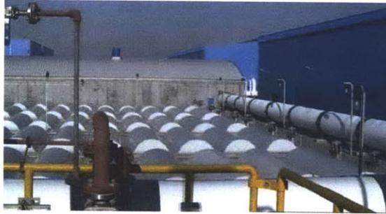
Figure 2: Close-up on the Multi-media filtration in Ashkelon SWRO plant. (photo credit to Sauvet-Goichon (7))
