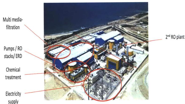
**Figure 1: Ashkelon SWRO plant. The multi-media filtration (on the left of the picture) requires a lot of space, are labour intensive and are associated with high capital costs. Chemical treatment can be more automatized but operation costs are still high, and anti-fouling membranes might lower the need of those costly pre-treatment (photo credit to Sauvet-Goichon (7))**
