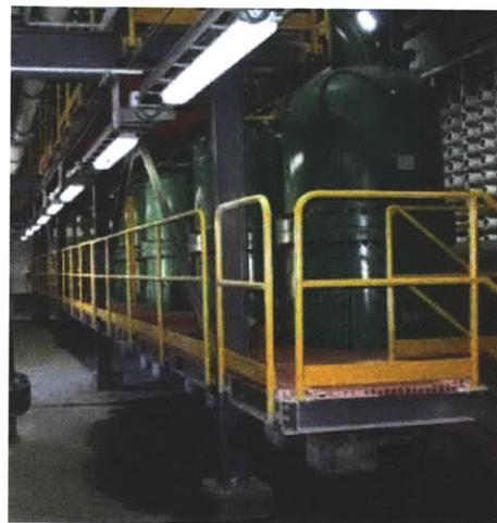
Figure 4: Cartridge micronic filters in Ashkelon SWRO plant. Micro-filtration is the last step to remove any particules (bio-foulants, agregates and colloids) above 1-5 $\mu$ m. (photo credit to Sauvet-Goichon (7))
