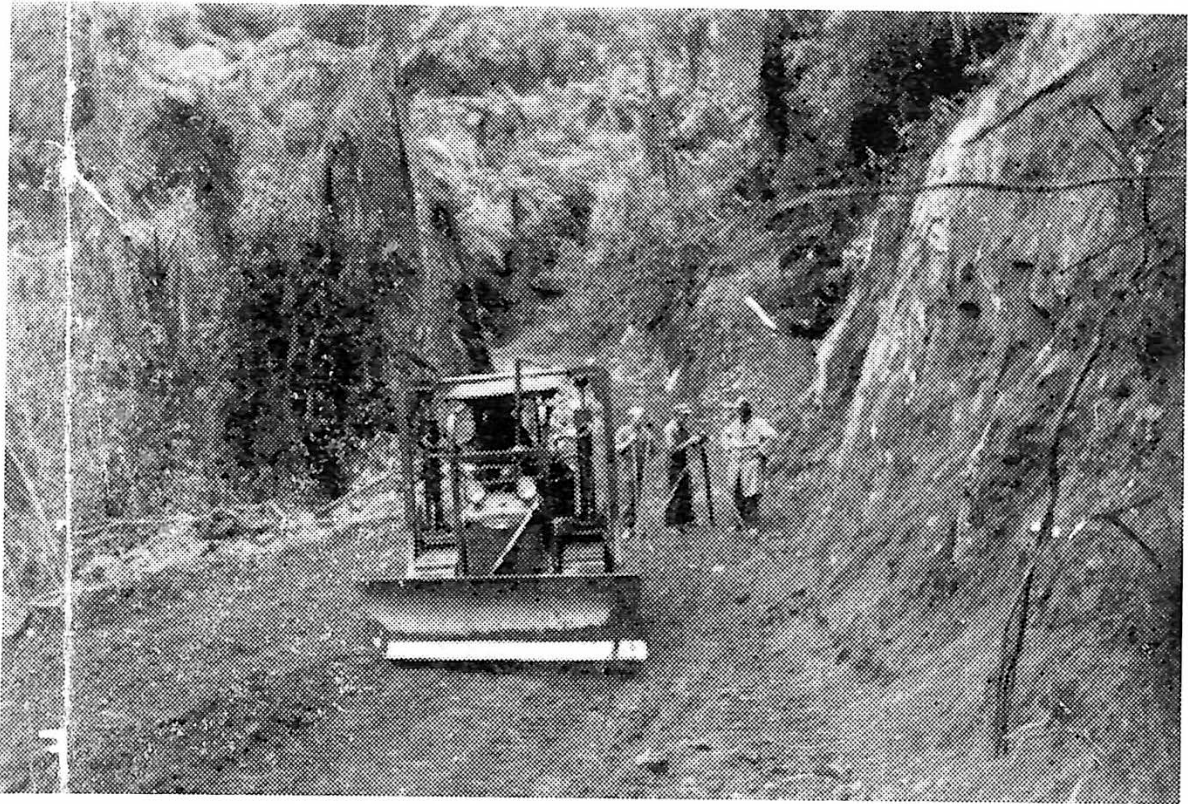
Figure 5: 'Excavating Site for Mine Buildings at 1600 feet'.
