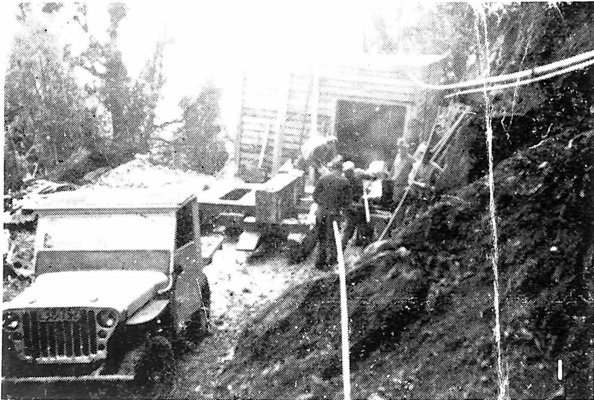
Figure 7: 'Preparing foundations for compressor and engine. "Jeep in foreground'.
