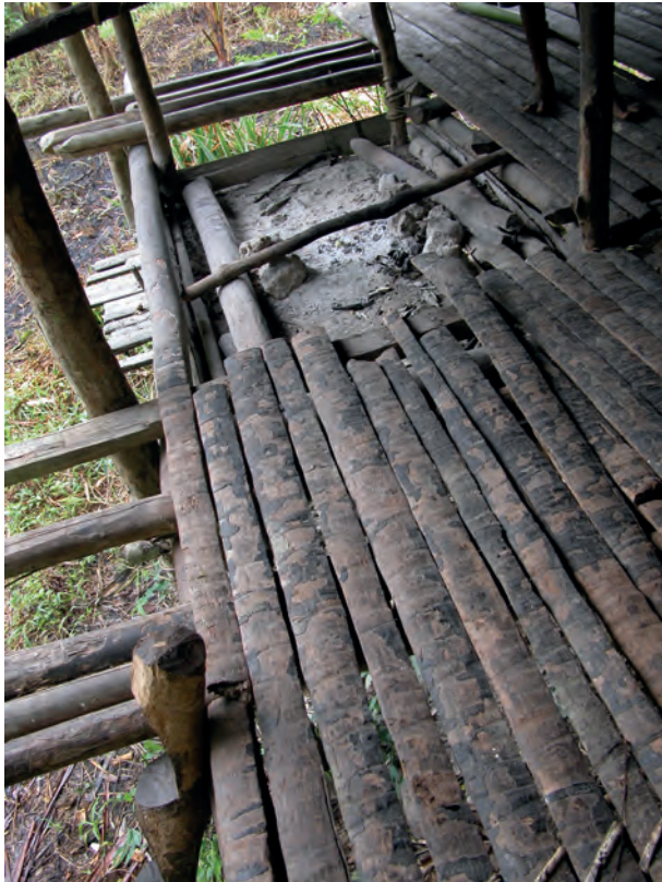
Figure 13 - Typical clay-lined fireplace within mid-Kikori River region stilt house, 2005 (photograph: Bruno David).
