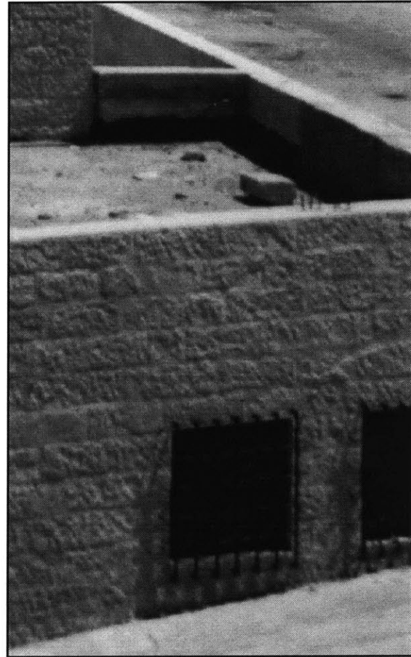
Figure 51. Use of metal bars on windows
