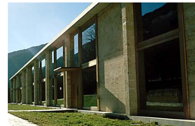
Figure 11: Home for Senior Citizens Graubünden, Switzerland Peter Zumthor 1993 An example of congregate housing
