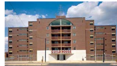
Figure 12: Guild house retirement home Philadelphia, Pennsylvania Robert Venturi 1960-1962 An example of congregate housing
