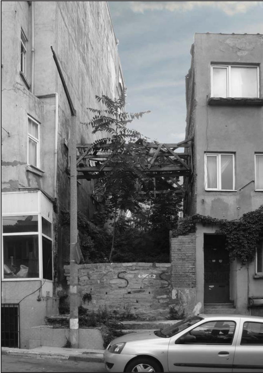
Figure 38: Trusses supporting partition walls. 68
