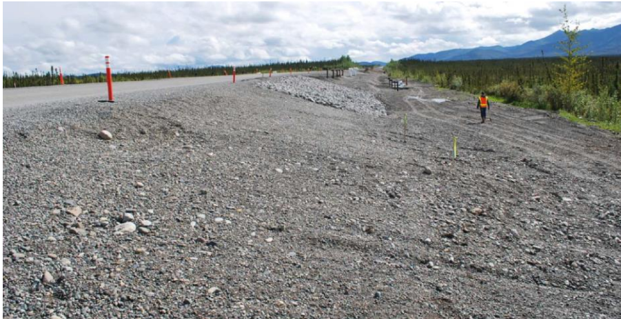
Figure A. 13: Snow cleaning technique (S10) after construction.
