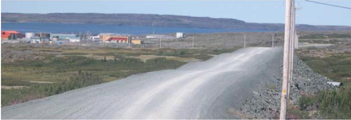
Figure 1. 6: Differential settlement.
