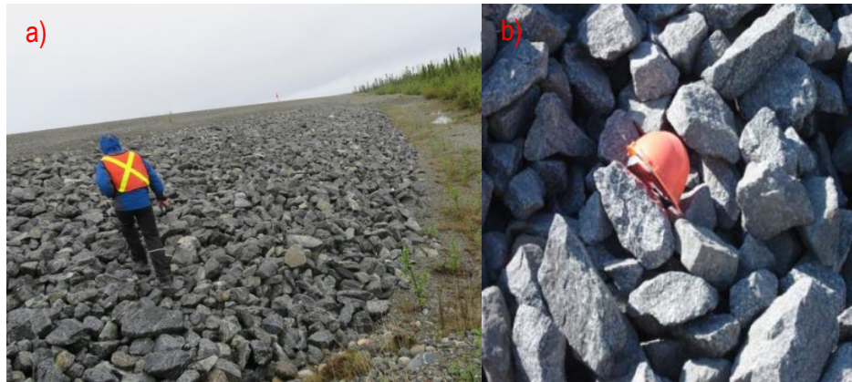
Figure 5. 2: The shoulder ACE section at Beaver Creek, Yukon. (a) General view; (b) Typical rock diameter.
