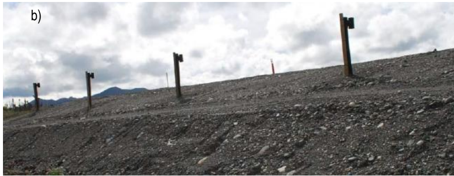
Figure A. 5: Heat drain across the whole embankment (S2) a) during construction; b) after construction.
