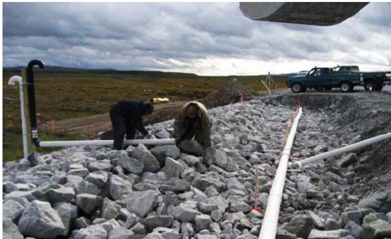
Figure B. 5: Construction of the air convection embankment (Doré et al., 2012).
