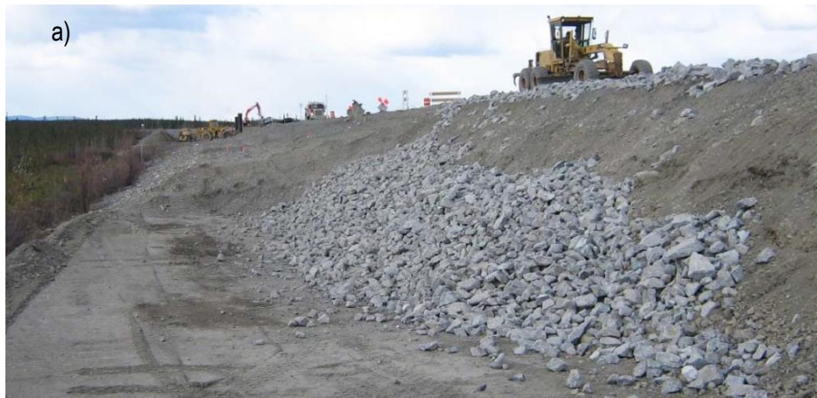
Figure A. 5: Heat drain across the whole embankment (S2) a) during construction; b) after construction.
