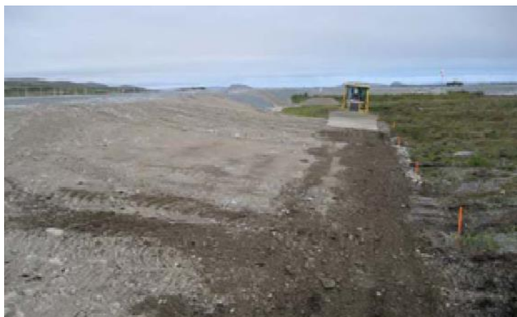
Figure 7. 2: Experimental gentle slope built on the Tasiujaq airstrip in Nunavik, Quebec.
