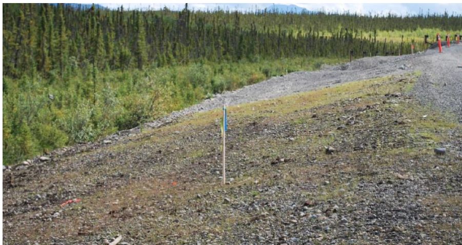
Figure A. 14: Grass-covered embankment on the side slope (S11) after construction.
