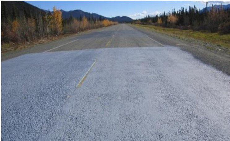
Figure 7. 6: High albedo surface with the cool gray colour on bituminous surface treatment (BST) on a test site on the Alaska highway in Yukon.
