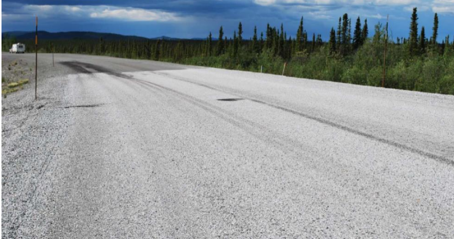
Figure A. 15: High albedo surface (S12) after construction.
