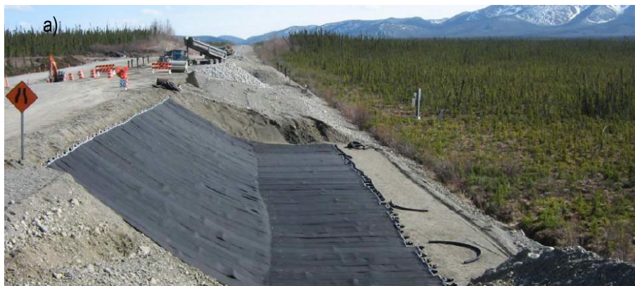
Figure A. 6: ACE on side slopes covered (S3) a) during construction; b) after construction.
