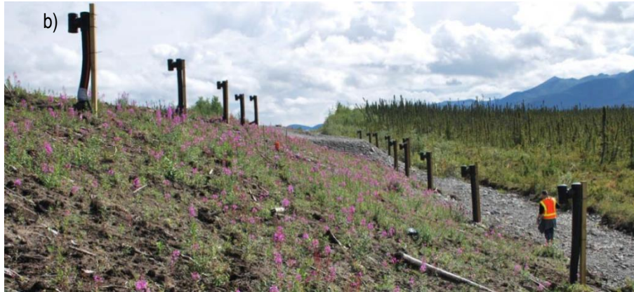
Figure A. 6: ACE on side slopes covered (S3) a) during construction; b) after construction.
