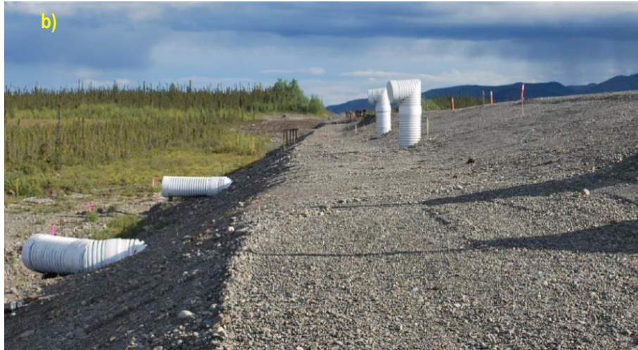
Figure A. 10: Longitudinal culvert (S7) a) during construction; b) after construction.
