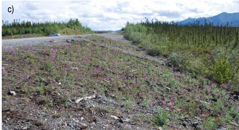
Figure 4. 2: Air convection embankment (ACE) at Beaver Creek, Yukon: a) diagram of the ACE; b) during the construction of the ACE; c) after the construction of the ACE.
