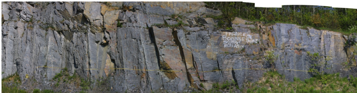
Figure 3: Scanline 1 (Fleurimont rock slope, May 24, 2007)
