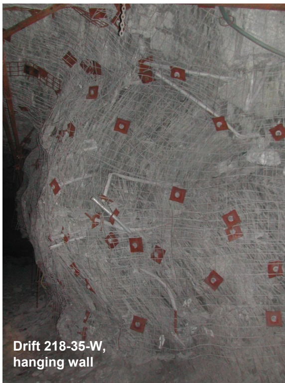
Figure 76: Rock support on level 218 and 227 (LaRonde mine, March 2008)
