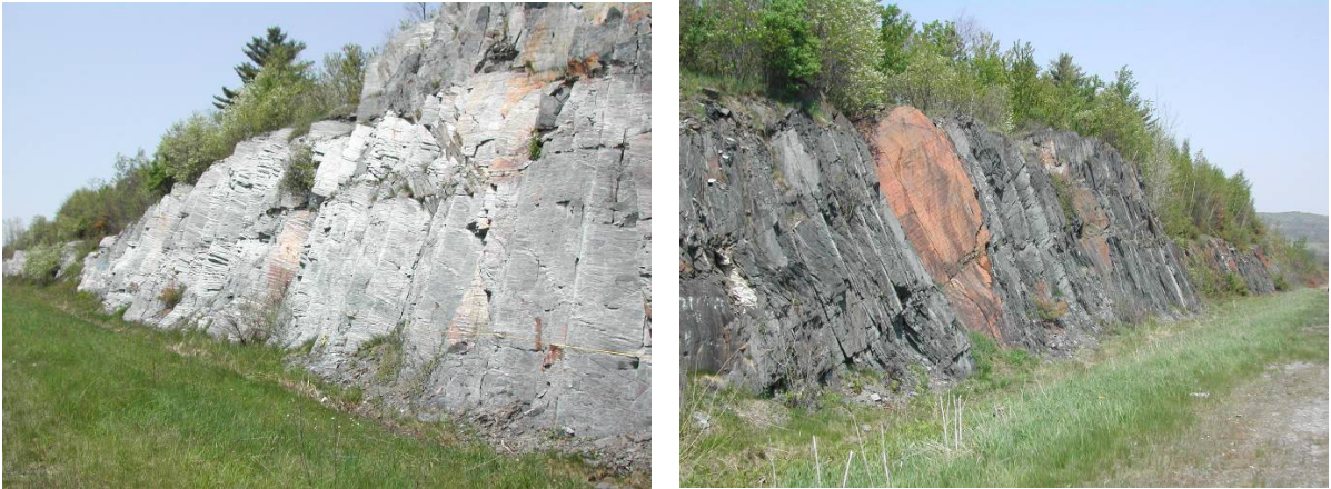
Figure 9: View along the Fleurimont rock slope in west direction (left) and east direction (right), May 24, 2007
