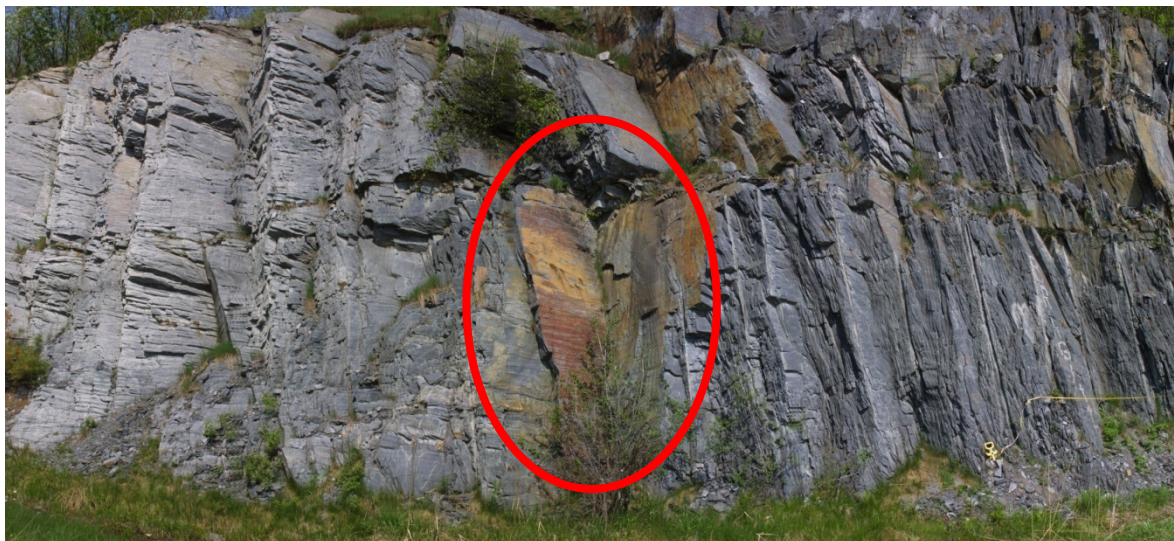
Figure 2: Investigated rock slope near Fleurimont with area of wedge failure (May24, 2007)
