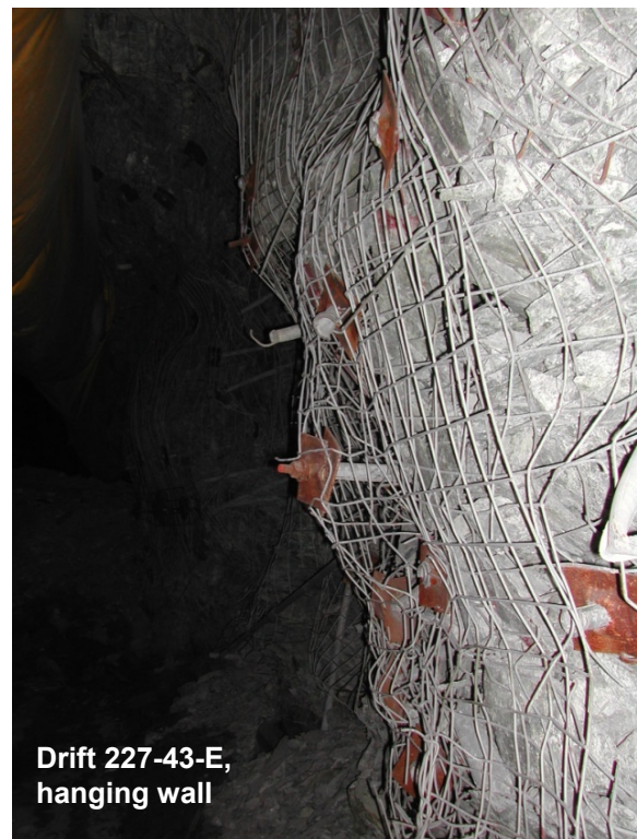
Figure 76: Rock support on level 218 and 227 (LaRonde mine, March 2008)
