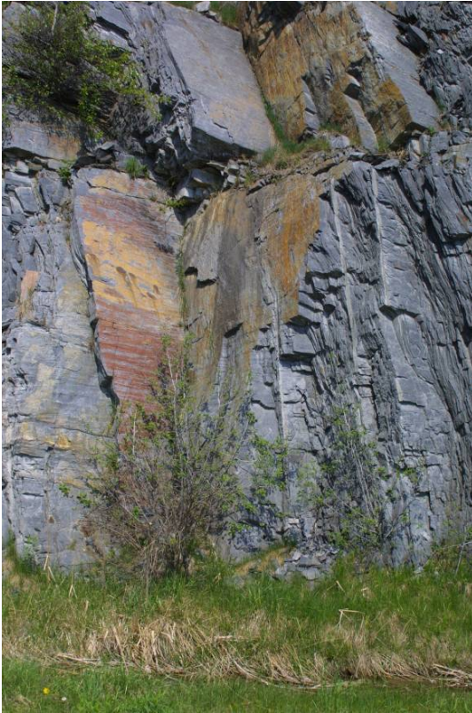
Figure 25: Wedge A (Fleurimont rock slope, May 24, 2007)
