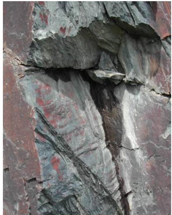
Figure 18: Water discharges out of joints (Fleurimont rock slope, June 07, 2007)
