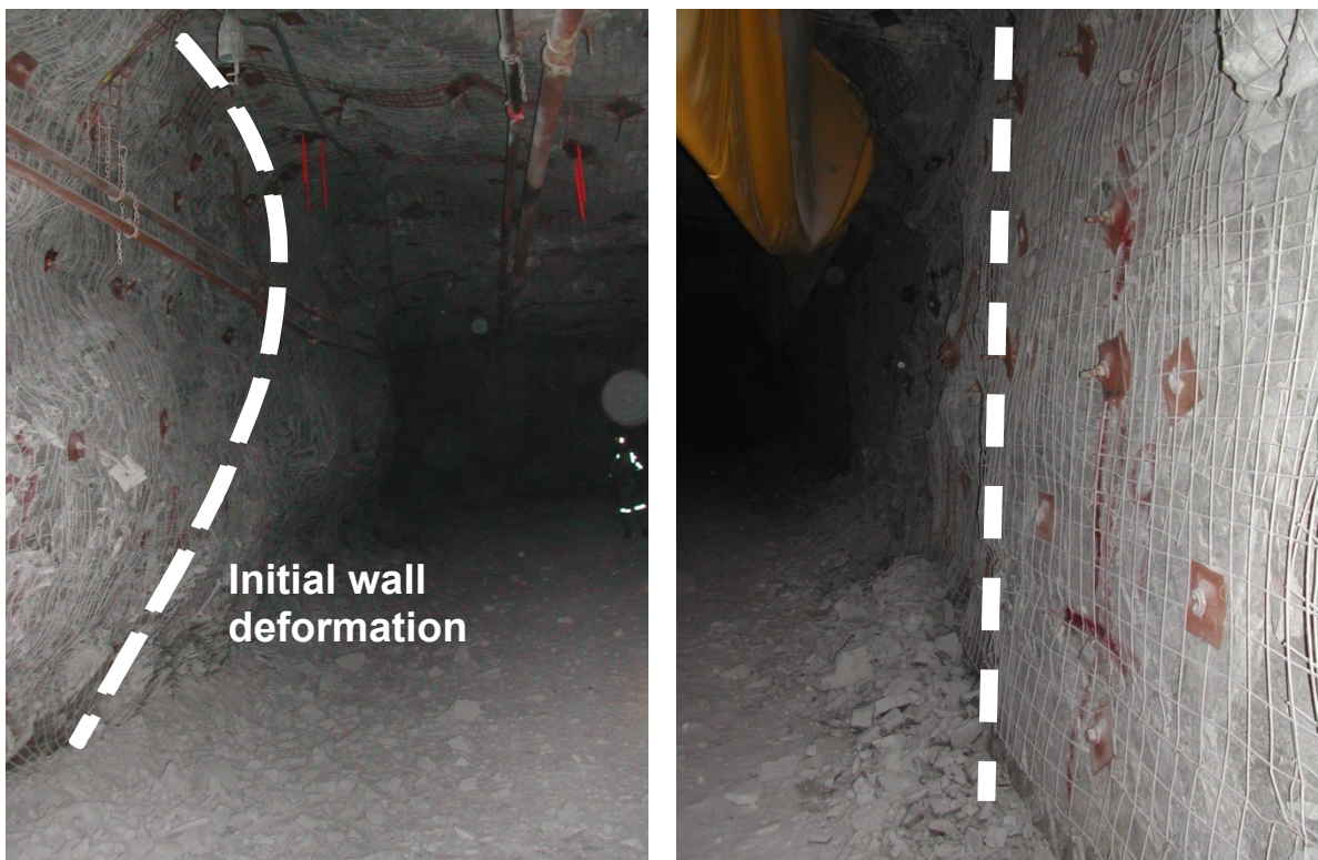
Figure 58: Hanging wall (left) and footwall (right) of drift 218-35-W (LaRonde mine, March 2008)
