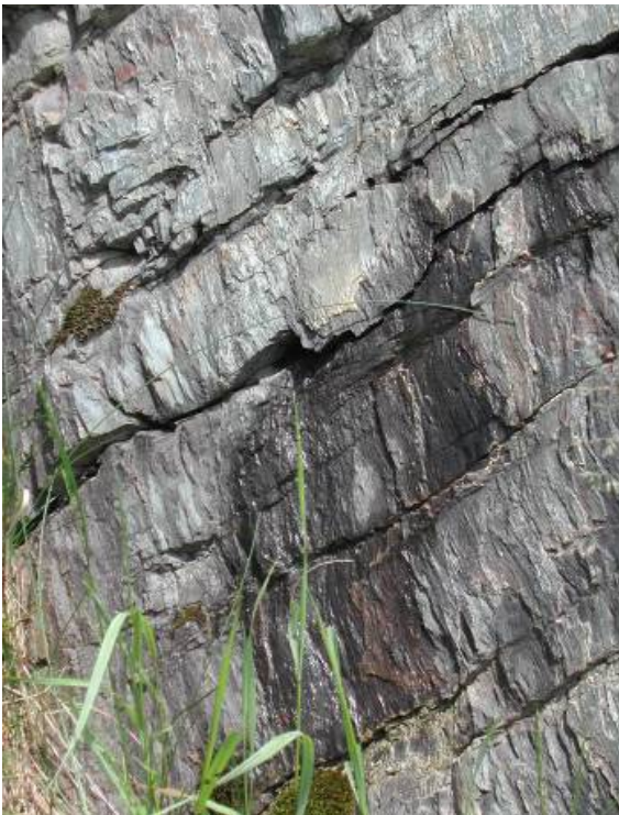
Figure 18: Water discharges out of joints (Fleurimont rock slope, June 07, 2007)
