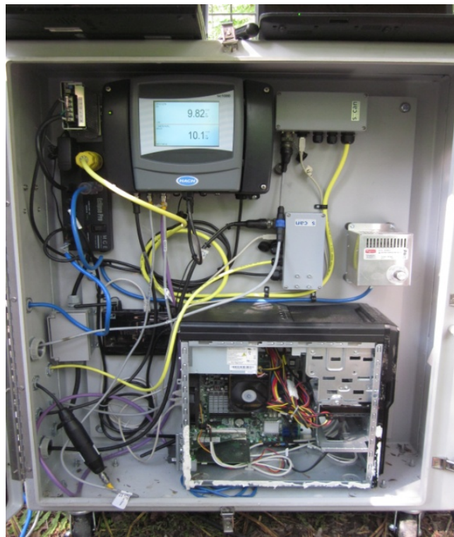
Figure 3 – The equipment panel of the monEAU monitoring station
