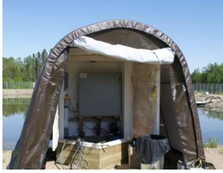
(a) Tent installed with a butane on the station's house at the inlet of the We-motaci F/AL.
