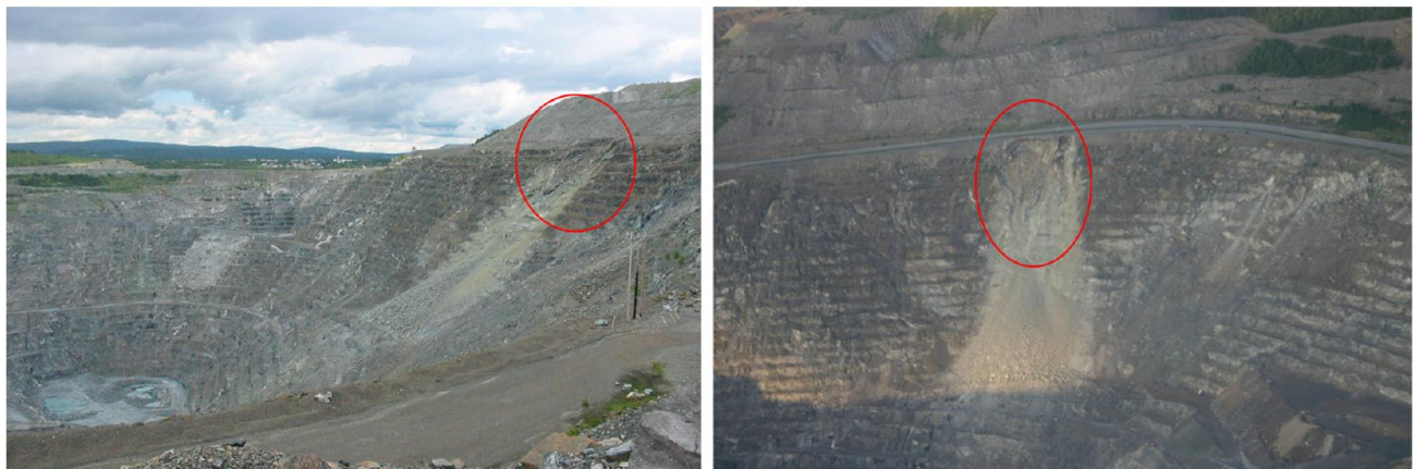
Figure 2. Early signs of failure on the evening of August 11, 2009
