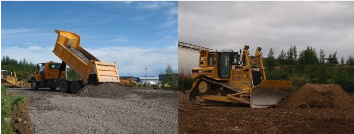
FIGURE 50 Building the foundation pad for the new greenhouse.
