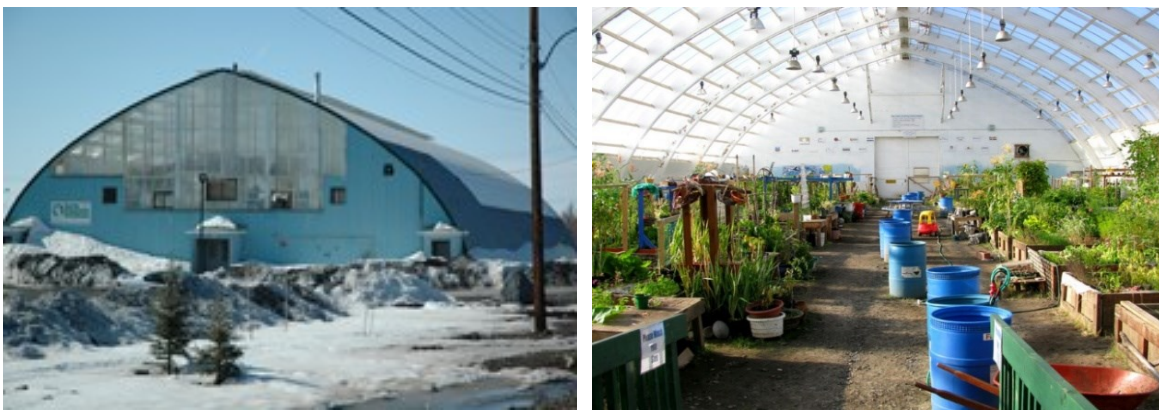
FIGURE 14 Exterior and interior views of the Inuvik Community Greenhouse.
