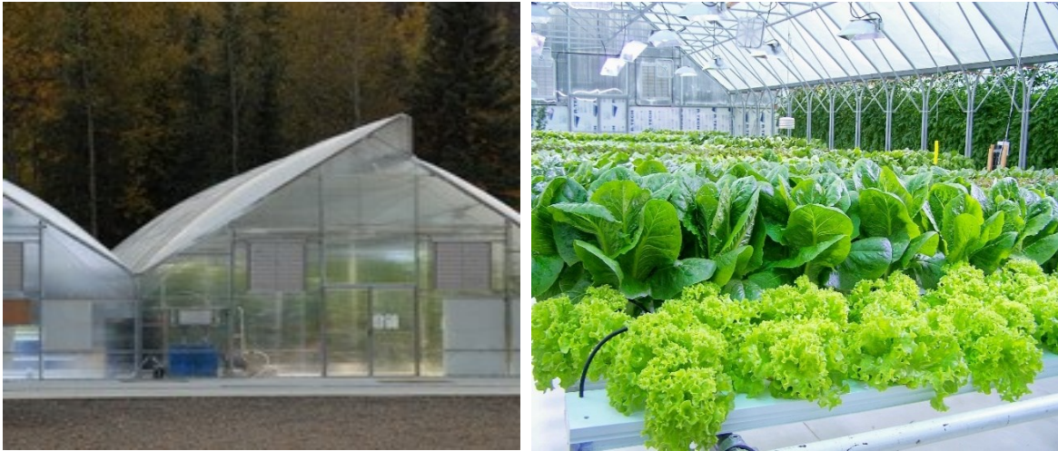
FIGURE 29 Exterior and interior views of the Chena Hot Springs greenhouse, Alaska.
