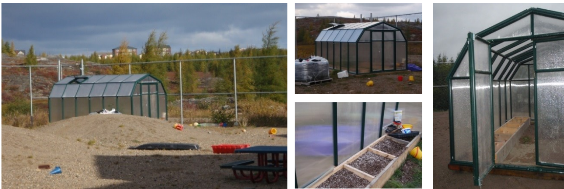
FIGURE 65 Interior and exterior views of new greenhouses installed at both daycares.
