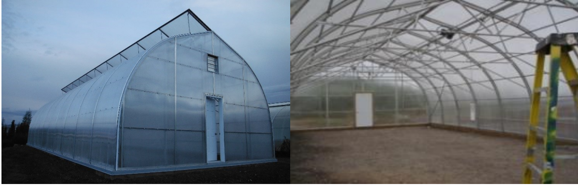
FIGURE 51 Exterior and interior of new greenhouse upon completion of construction.
