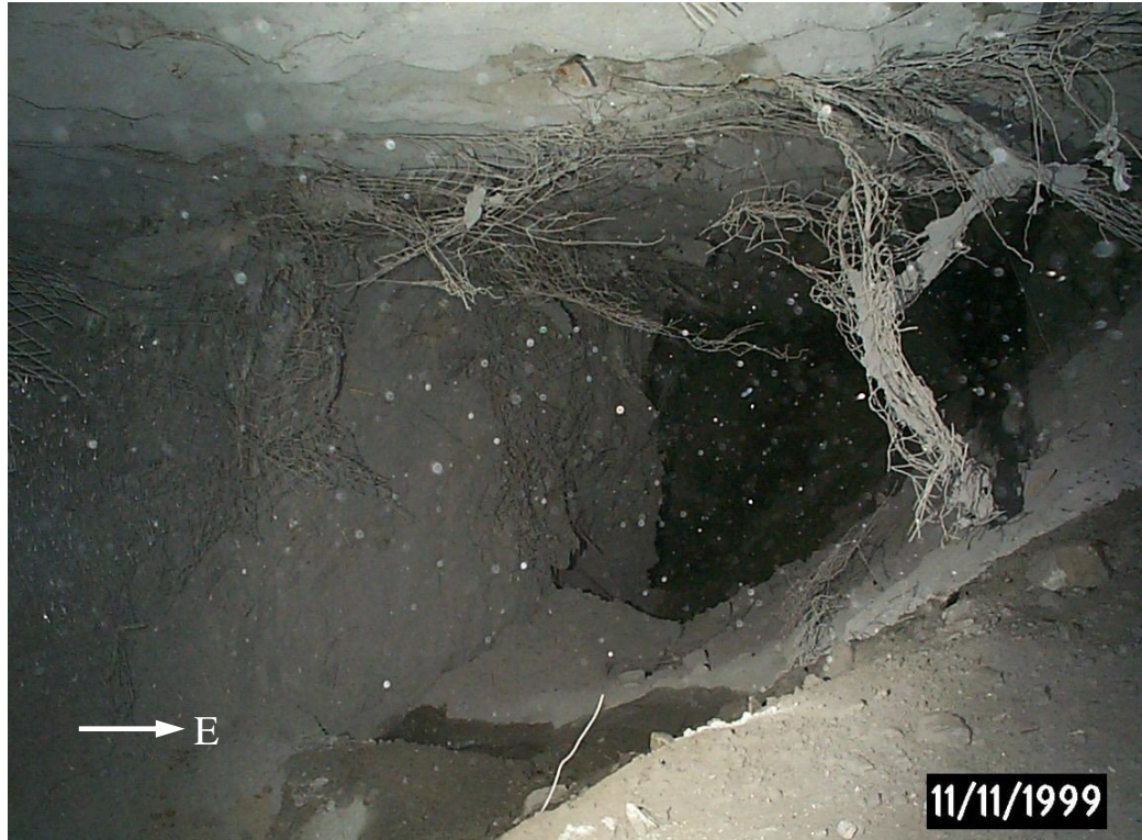
Figure 69. Photograph looking north in the 29-9 Pillar overcut on 1000 Sill. This picture was taken further north from the area depicted in Figure 68. (After Andrieux et al. , 2000.)
