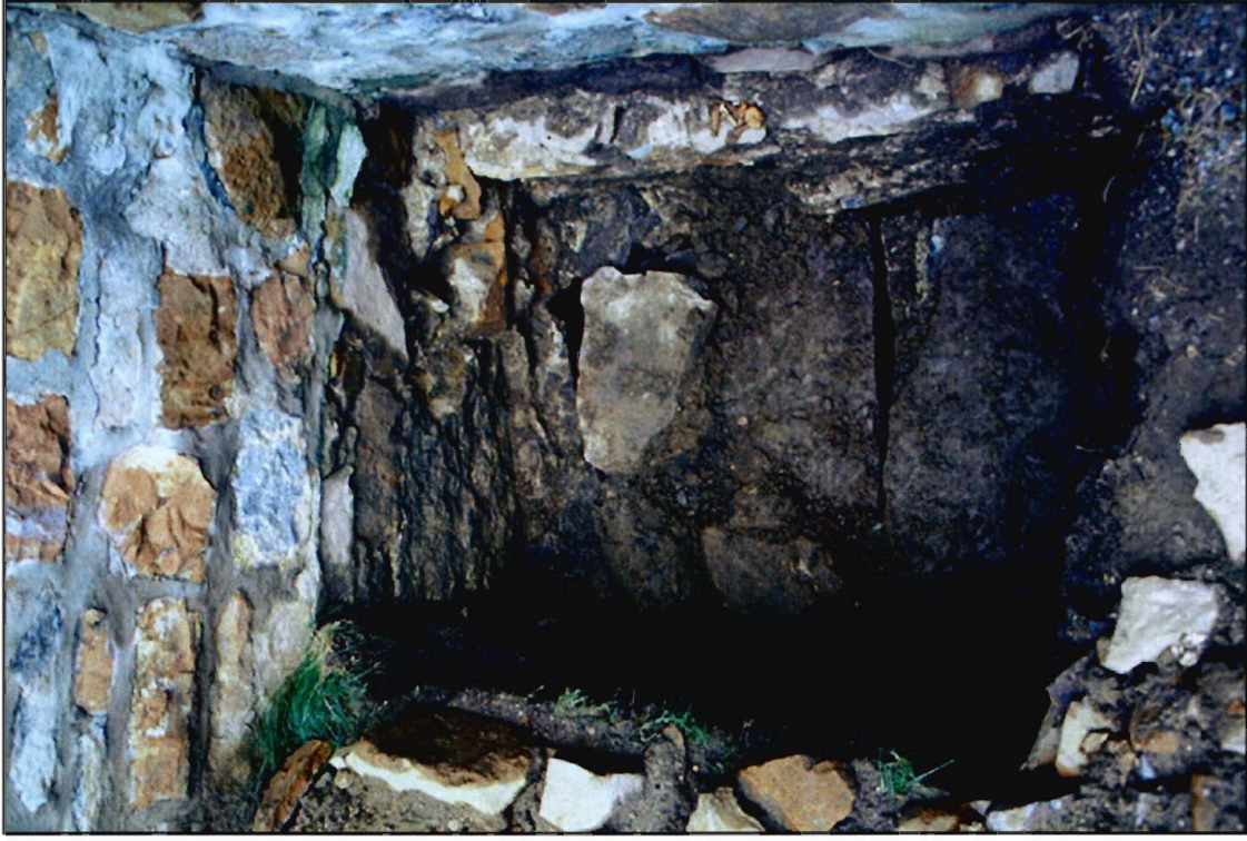
Figure 73 : Drain 10F9 (BjFj-84-01-D3-25)
