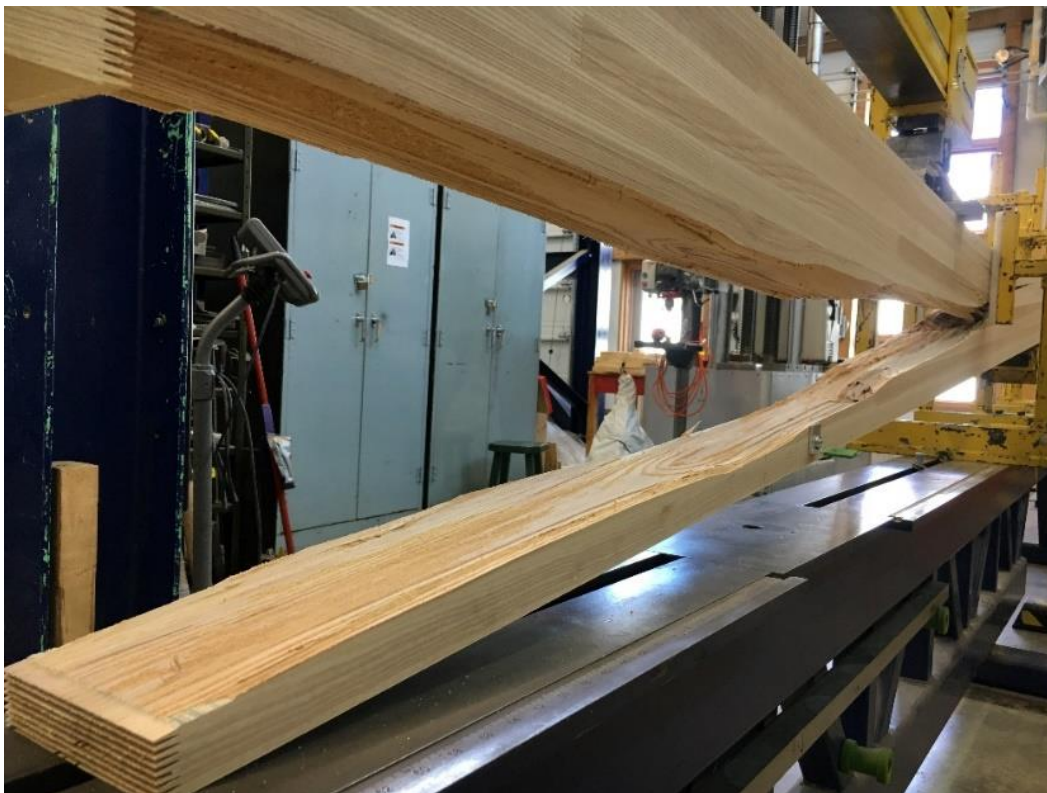
Figure 21. Failure of a white ash glulam beam initiated at a finger joint.
