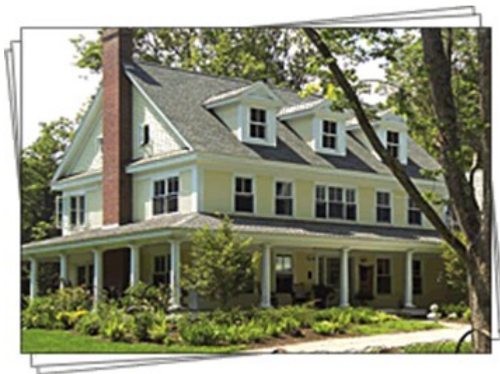
Figure A.2. Building with UV-resistant coatings (Maibec Inc., Québec, Canada).
