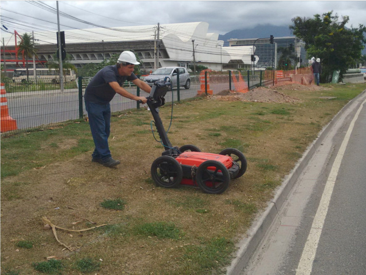
Figure 3.2: Ground-penetrating radar survey in progress.
