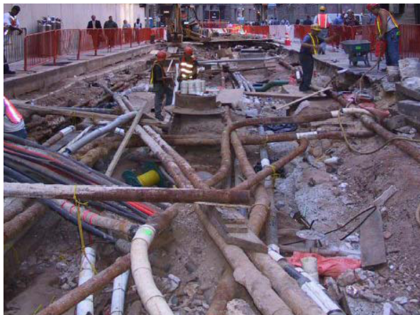
Figure 4.1: Example of underground utility networks, Rio de Janeiro (Courtesy of Geovoxel).
