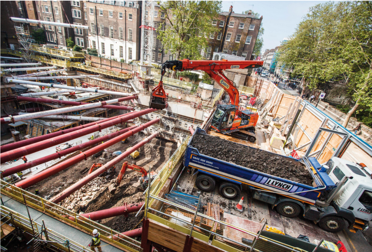
Figure 3.1: Example of underground utility networks, central London. Image courtesy of Hitachi (Source: Bentley Intelligent 3D Models).
