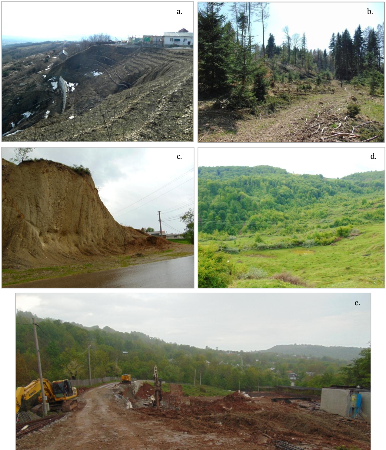
Figure 8. Space planning limitation issues in Cămpinița Hills. a. Engineering works on a complex landslide body affecting Cornu Monastery, in Cămpinița Basin (January 2015); b. Deforested area on the Prahova – Cămpinița interfluve (April 2015); c. Steep-slope above the DJ 207 road in Șotrile village (May 2015); d. Humid grounds on the hill slope, generated by the moving mass of the landslides (May 2015); e. DJ 207 road affected by a landslide in Vistieru village area (May 2015).
