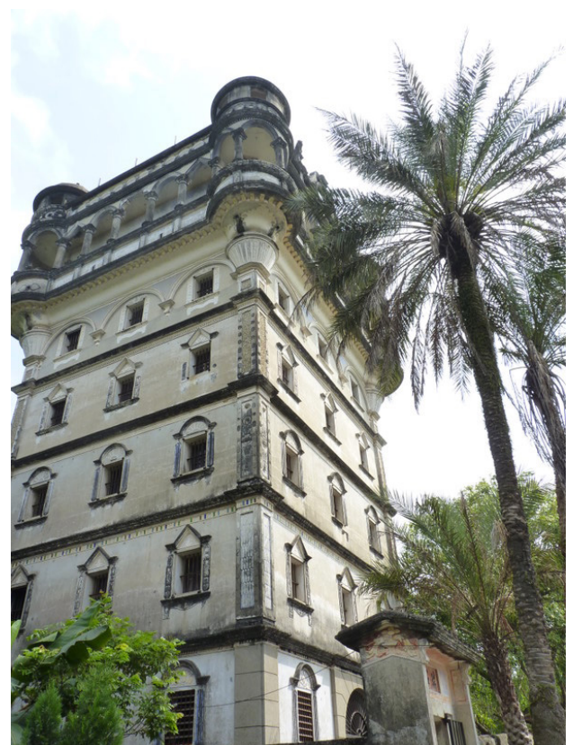
Figure 9. Ruishi Lou in Jinjiangli village (source: field survey)
