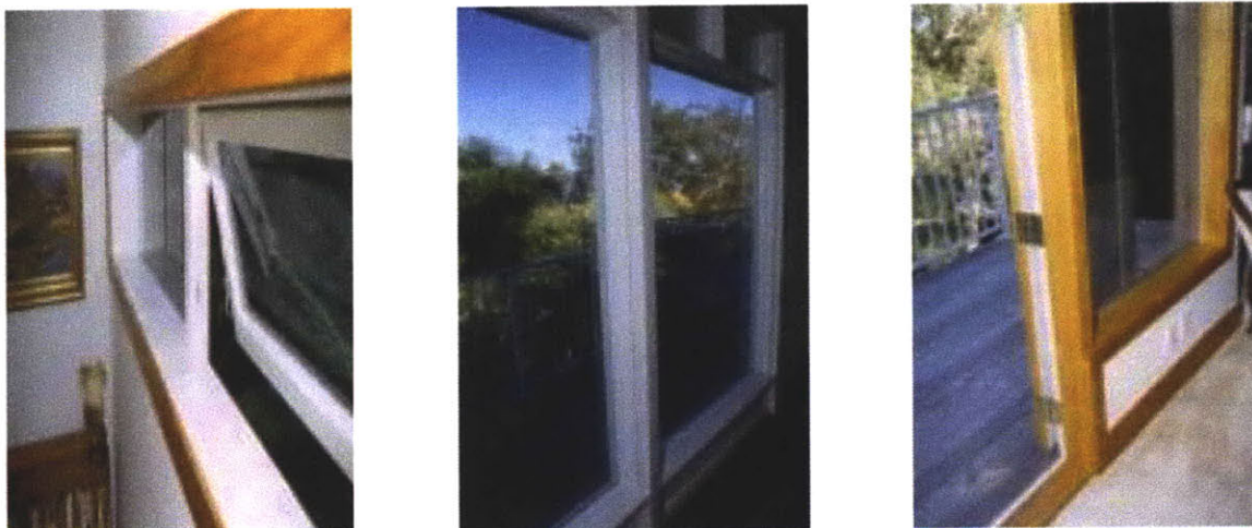
Figure 19: (From Left to Right) Reused, Retained, and New Windows (Storey, p. 108)
