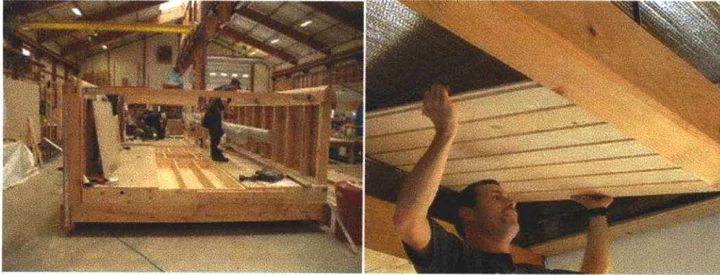
Figure 18: Assembly of Interior Walls and Ceiling Panels (Dey, pp. 60-61)
