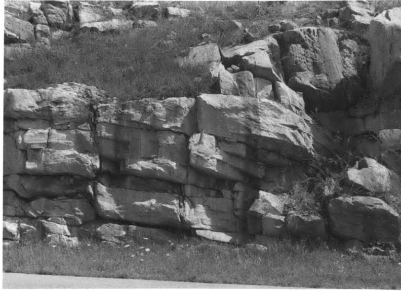
Figure 3.- Steeply-dipping grayish green dolomite, calc-dolomite, and schistose dolomite of Unit 2-G. Note weathered surface in contrast to fresh surface. The shallow-dipping north-south joints normal to the compositional banding is presumably associated with the Sherman Hill anticline. Two miles south of Dover Plains on Route 22 - Locality 24.
