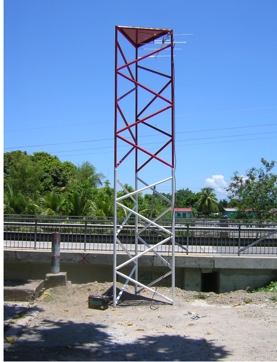
Figure 4.11: 5 Meter Antenna Tower for Radio Nodes at Saba
