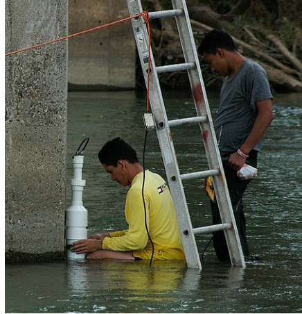
Figure 4.12: Installation of Water Level Prototype by FSAR Employees
