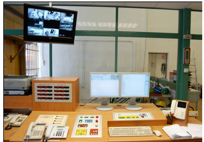
Fig. 1. Human-machine interface of the VR-1 reactor (before HMI desk upgrade in mid-2018)
