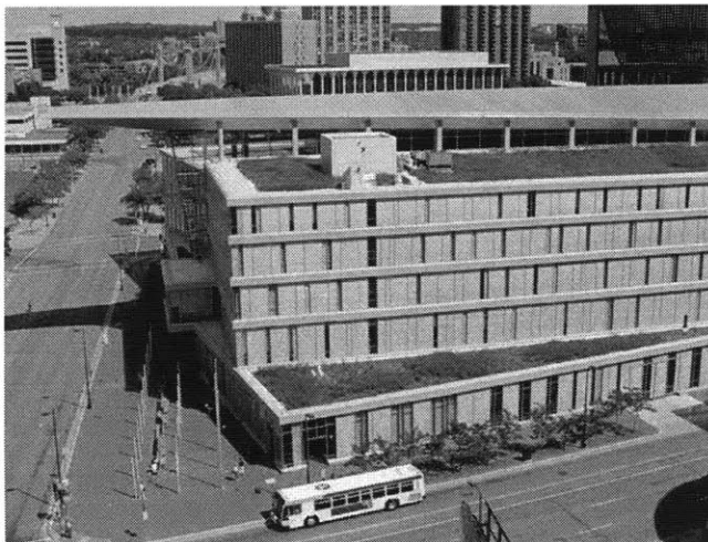
Minneapolis Public Library green roof
