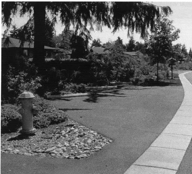
Angled parking and vegetated swales adjacent to a narrow residential street with flush curb
