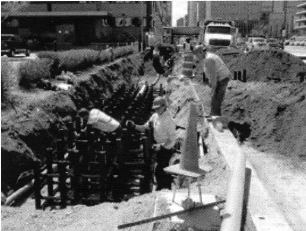
Photo: Installation of Silva Cell frames for street tree plantings (Anon. 2010)
