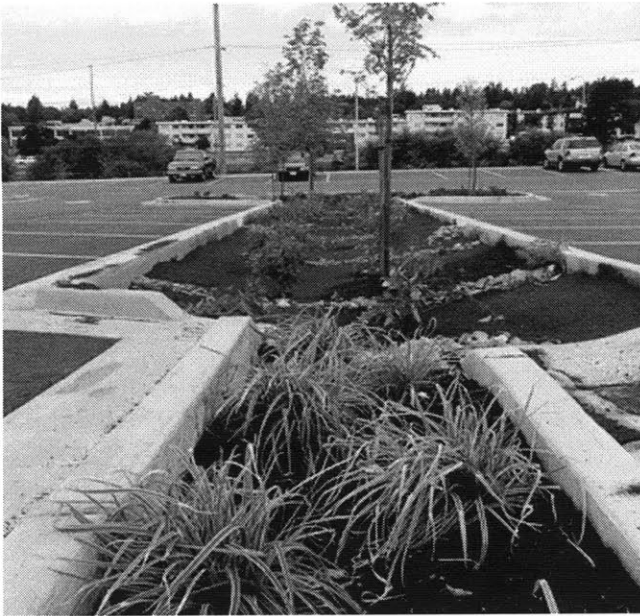
Northgate green parking lot
