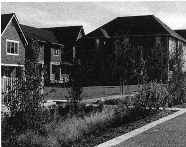
Streetside bioretention swales at High Point Development
