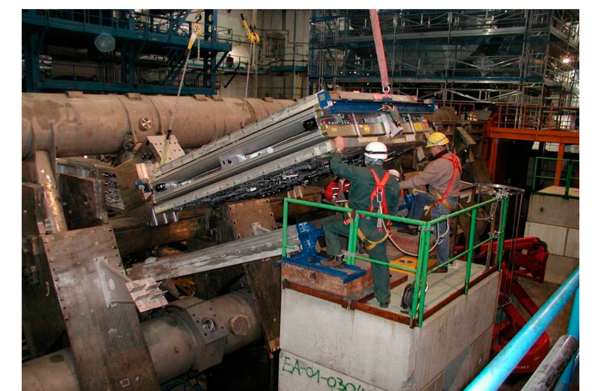
Installation of a barrel chamber
