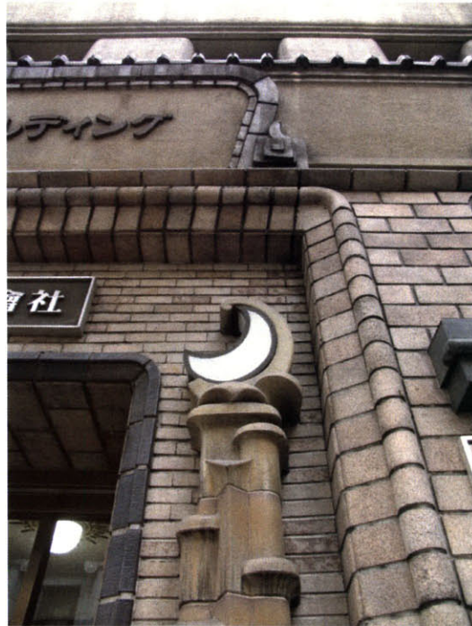
Figure 5.5 Ornament Details of Kourabashi Nomura Building Photograph taken by author.
