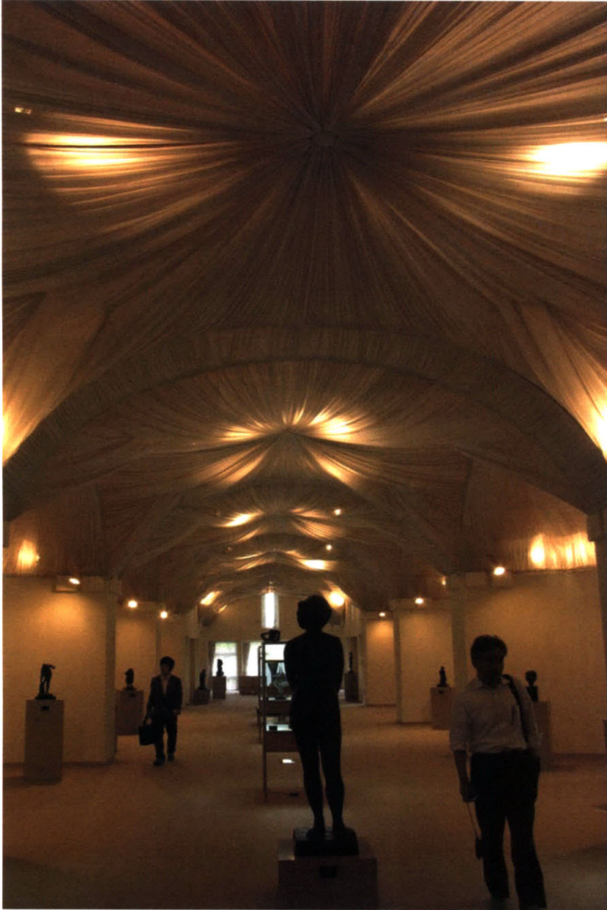
Figure 5.18 Interior of Yatsugatake Art Museum (1979) showing the fabric covering the ceiling. Nagano, Japan Architect: Murano Togo Photograph taken by author
