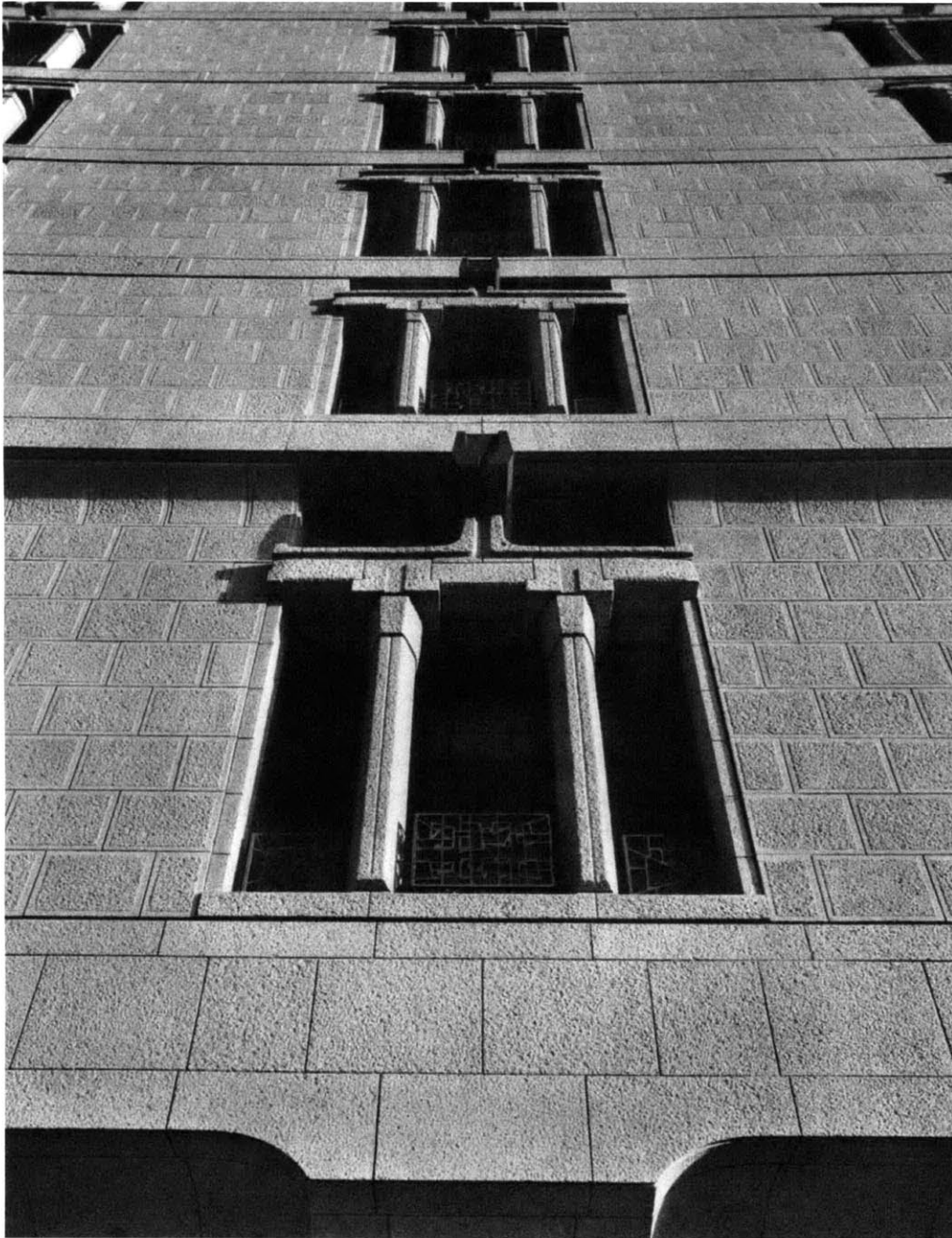
Figure 5.14 Wall details of Nissei Hibiya Building showing granite stone panels. Murano Togo Sakubin shu vol-1 - 232
