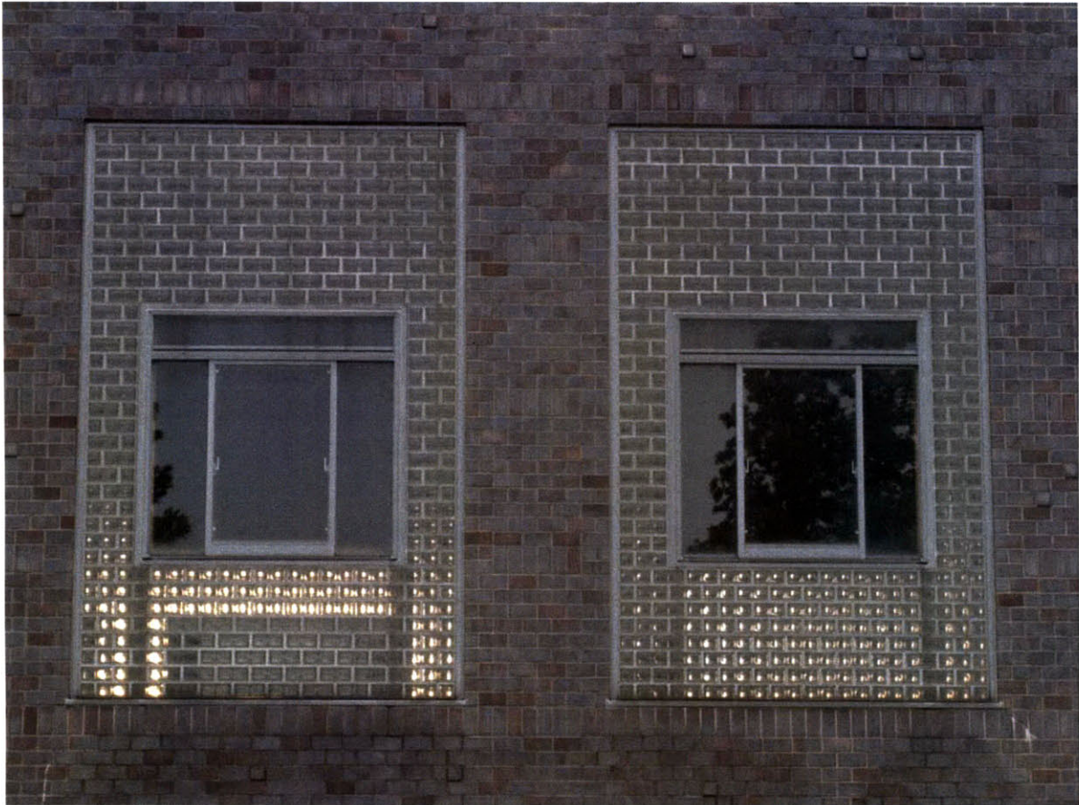
Figure 5.13 Wall details of Ube Civic Hall showing glass blocks and tiles. Photograph taken by author.
