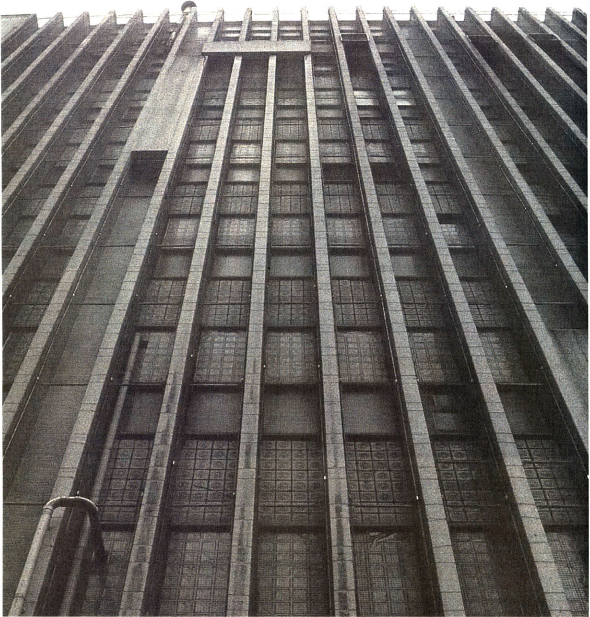
Figure 5.24 Sogo Department Store Close up view of façade Murano Togo Kenchikusekkei Zuten Katalogu vol - 3 - 4
