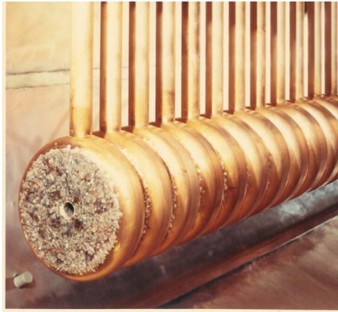
Figure 1. Initial drift tubes in the Los Alamos DTL showing arcing damage.
