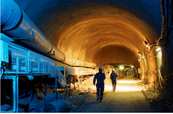
Figure 1.4: The excavated and bare LHC tunnel.
