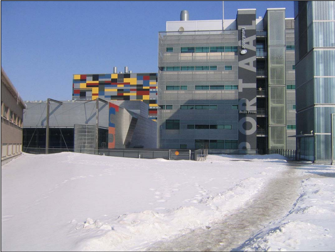
Figure 4.2: Dense mix of uses in Arabianranta: A factory, the University of Art and Design, and the Portaali Business Park are directly adjacent to each other. Source: Photograph by author
