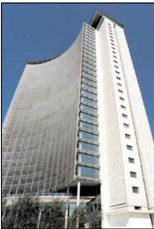
Figure 3.5: Exterior view of Empress State. Source: Landflex
