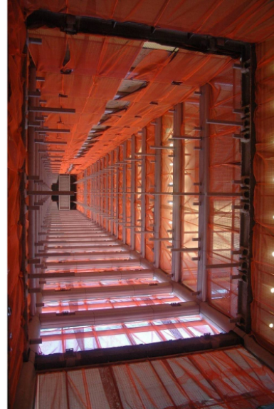
Phase 2 Elevators Under Construction in Atrium Space
