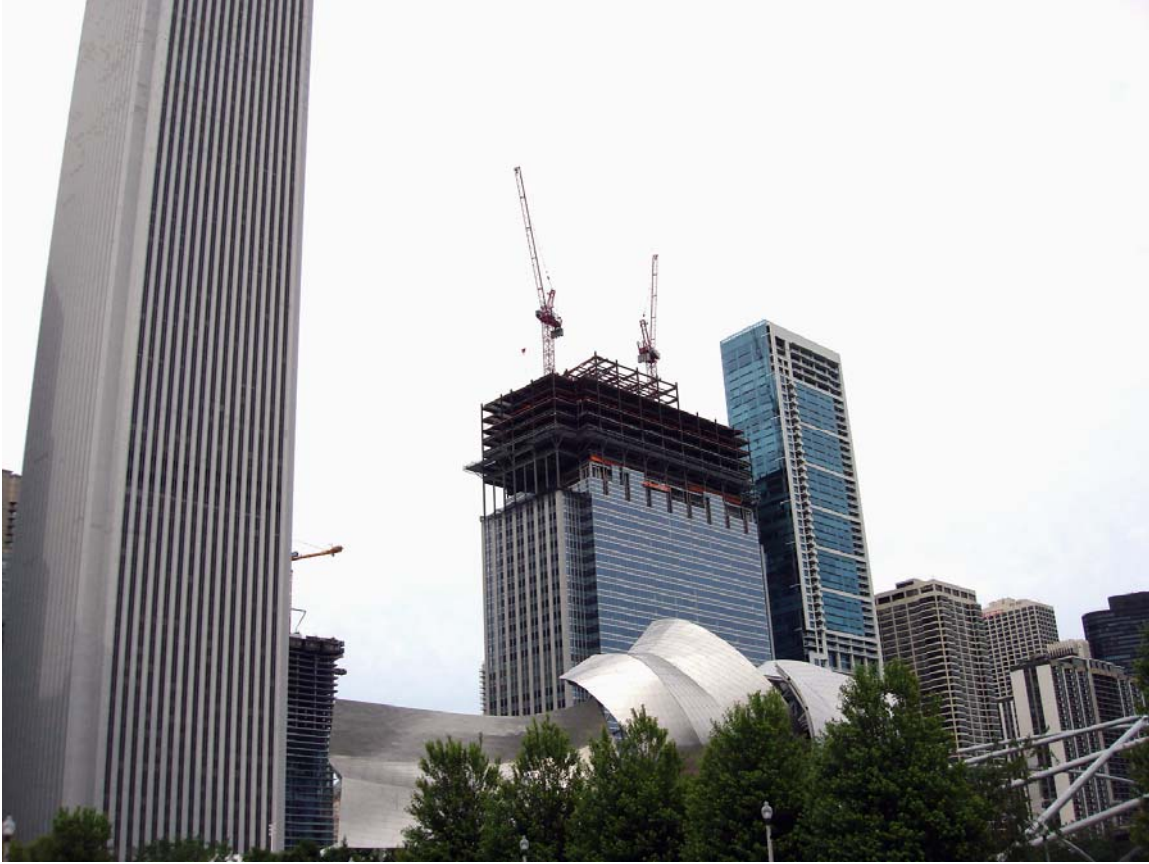
Figure 1.1: HCSC headquarters with vertical expansion / completion seen under construction, 2008 (Source: Author).
