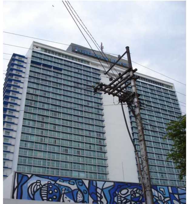
Photo 7: Exterior of Habana Libre Hilton. Photo taken by Damien B. Chaviano on June 22, 2008.
