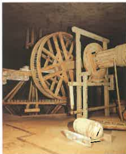
The Modena Chamber A horse gear used for vertical haulage
