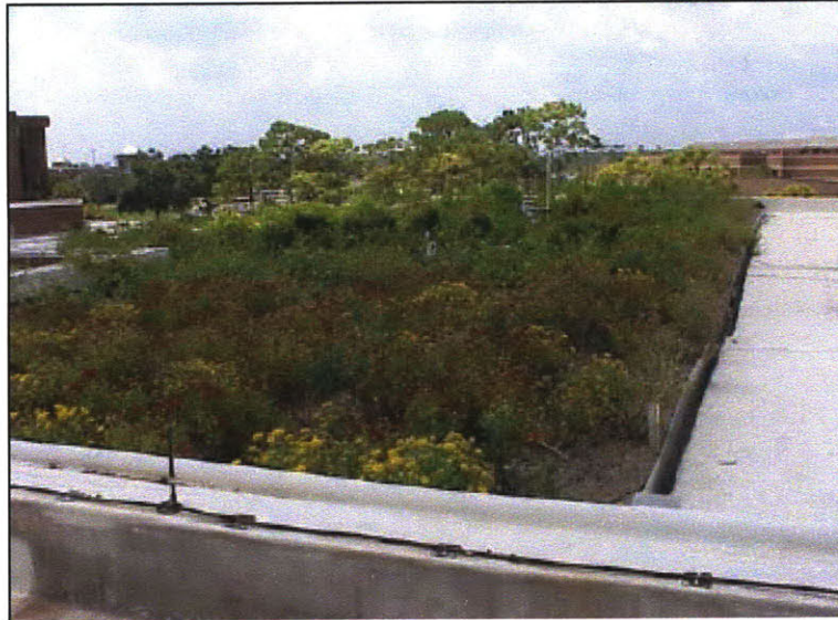
Figure 2-14: The extensive green roof with native Florida vegetation up to 2 ft in height, planted in 6 to 8 in of plant media. The conventional light-colored membrane roof is visible on the far right of the picture [35]
