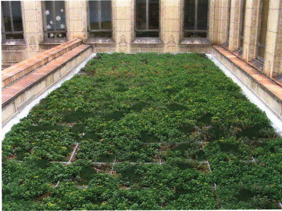
Figure 1-13: An extensive green roof in New York, New York. Source [14]
