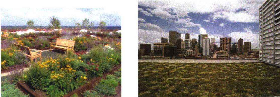
Figure 1-15: (left) An intensive green roof, characterized by heavier structural loads, high capital and maintenance costs, and accessibility to occupants. (right) An extensive green roof, characterized by lower capital and maintenance costs and lighter structural loads. Source [64] [38]
