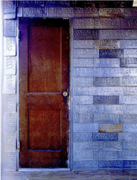
Outhouse, Newbern, AL | 1998-2001 Sheathing made of licence plates
