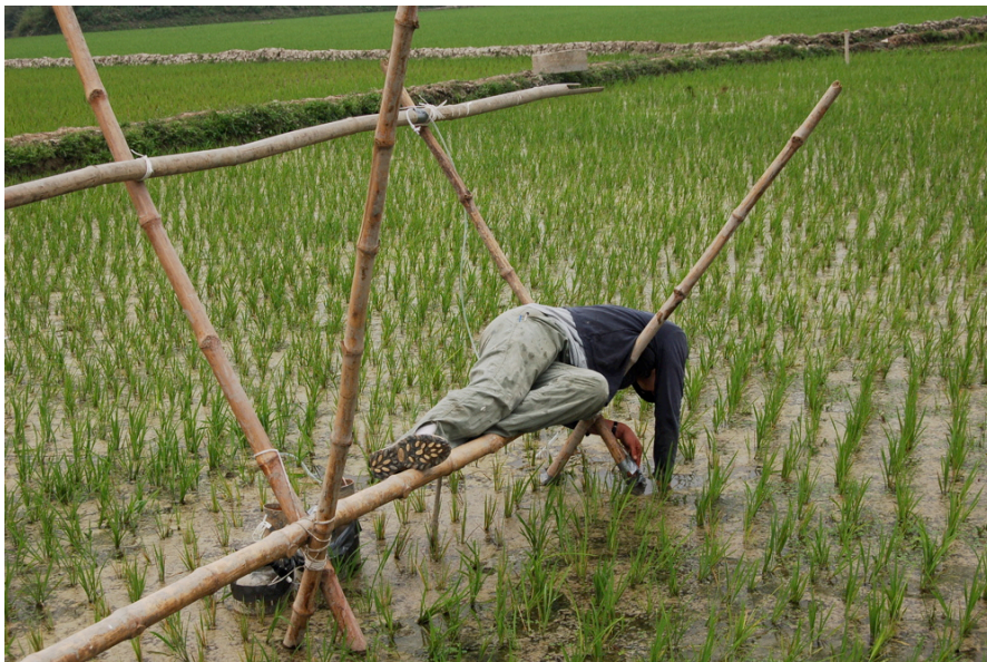
Figure 5.3 Close up view of bamboo scaffolding at location (e).
